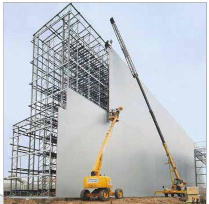
**Special systems** for pallets, containers and drawers composed of racks and software-driven travelling lifts, that plan the picking and the storing.
