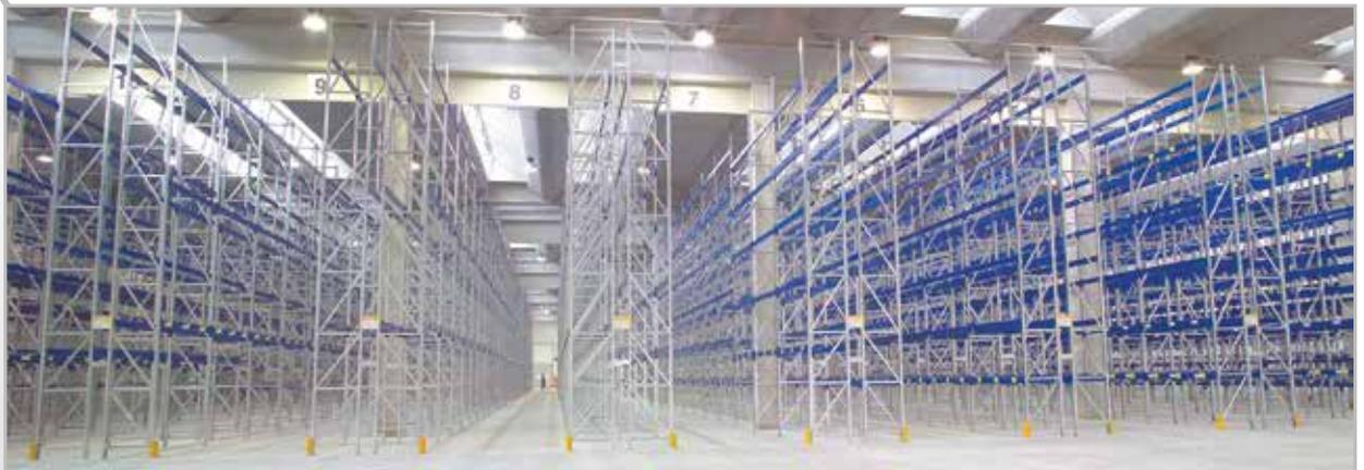
*The pallet racking system is the most traditional system for the easy store. The dimensions are determined according to the used truck and to the characteristics of the charge units.*
